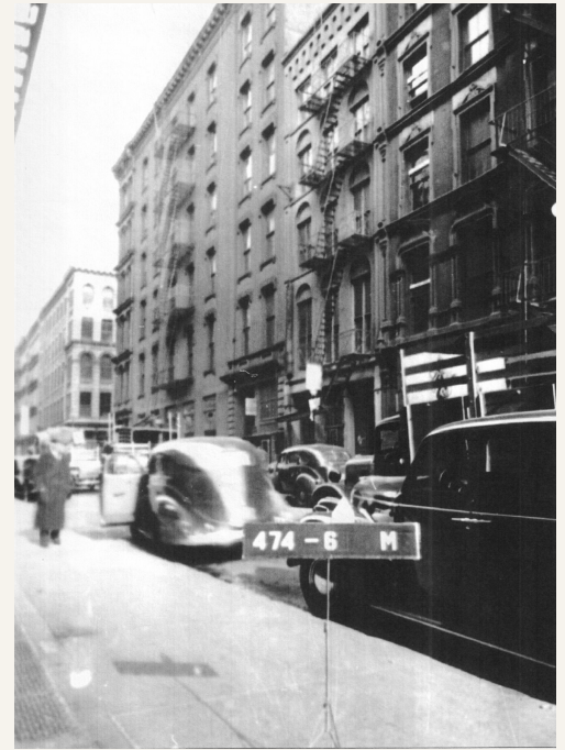
Greene Street storefronts, 1940s
